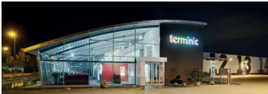
Terminic gained second place in the awards presented by a German trade magazine for the most attractive production plant
