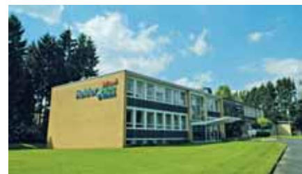
An 18,000m 2 plot of land acquired in the 1950s offers plenty of room for further growth
